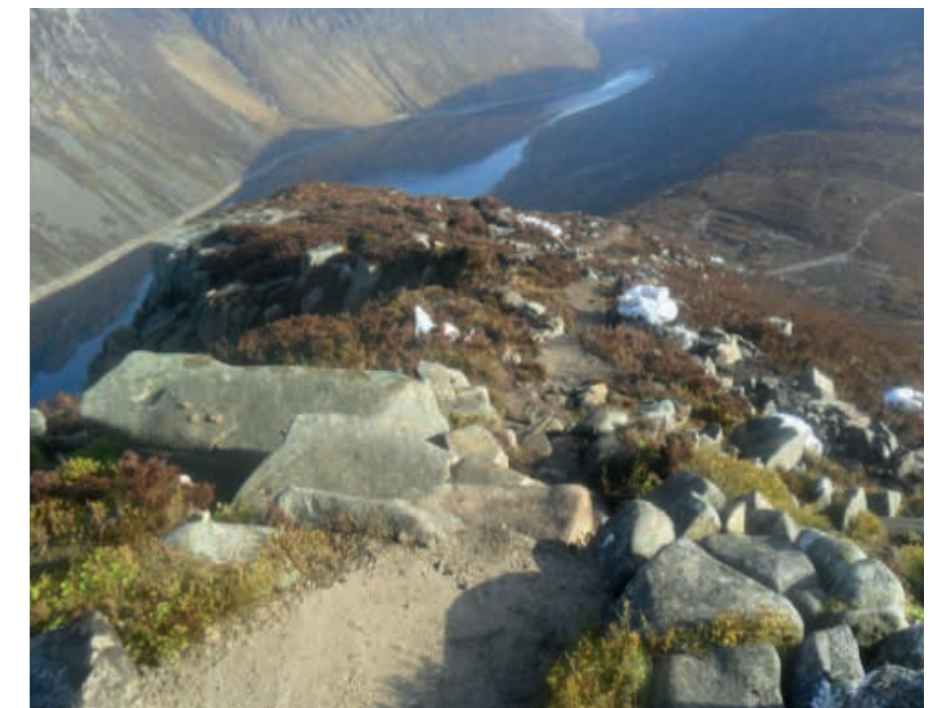
Upland Path Works on Binnian Mountain
